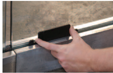
Adhere TAPER-LOC® L-Setting Blocks to the bottom edge of glass.
