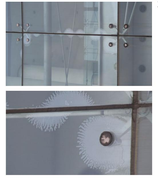
Typcial defects caused by delamination.
